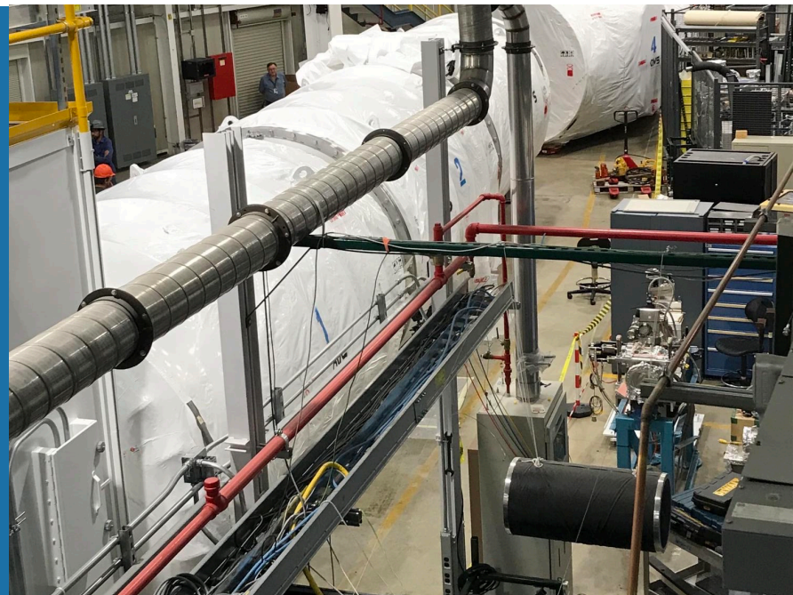
CSSI Grand Tube installation at 9-ID
