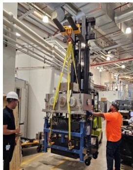
4-ID primary mirror installation
