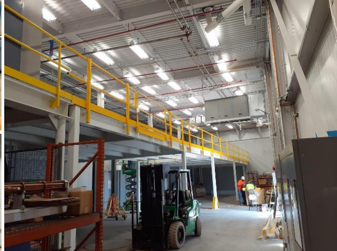
400A mezzanine structure near complete in Sept 2020
