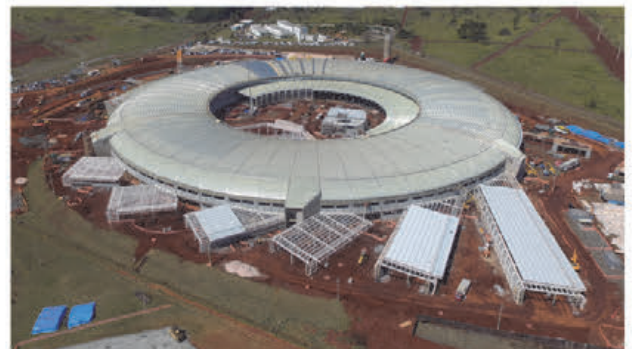
Figure 4: Aerial view of the Sirius construction site in August 2017.
