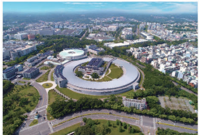
Aerial view of TLS and TPS rings
