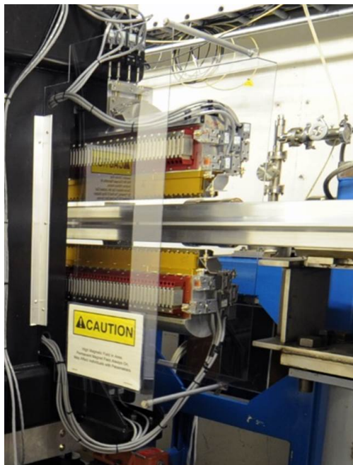
Figure 5.51. Revolver undulator installed in sector 35 in the current APS storage ring.
