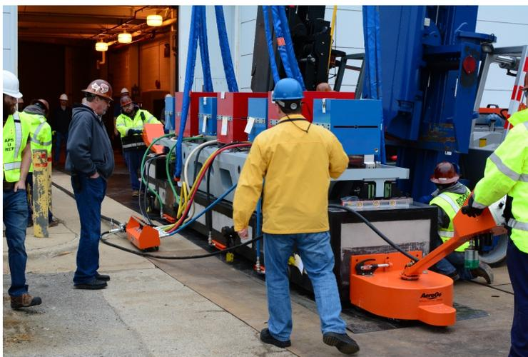
*Figure 4.144. Prototype FODO module being moved into the test area using an air caster system after it was unloaded from a flatbed truck using two Versa-Lifts in tandem.*
