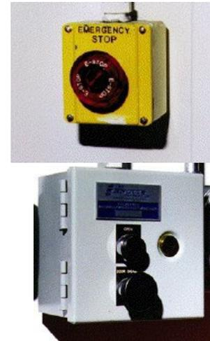
To open a pneumatic station door that has a magnetic locking system and leave the station, push and momentarily hold the DOOR OPEN button--automatic doors should slide open. If the door does not automatically open at that point, push the DOOR DISABLE button, which will dissipate any remaining air pressure. You will then be able to push the door open.
