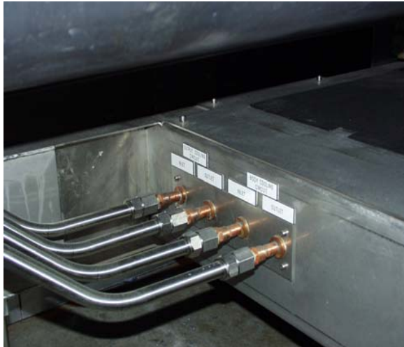
K3513A body and output Cavity inlets and outlets
