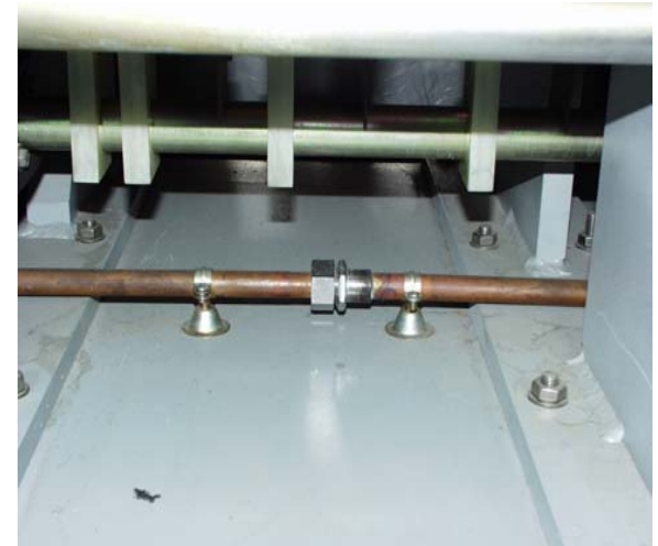
TH2089A body-1 water circuit
