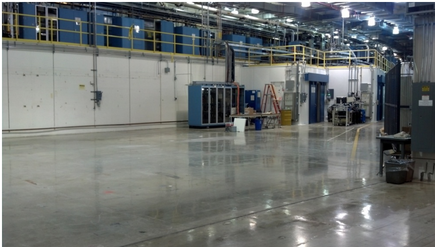
Preparing for construction at Sector 35
