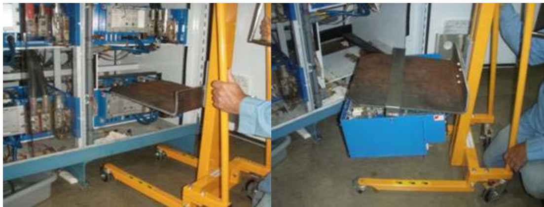
Lifting of storage ring power converters.
