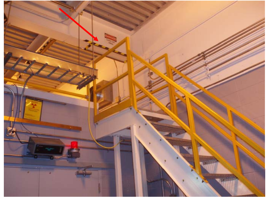
The staircase is located at building 420 RF test stand.
