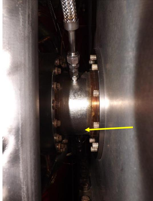
Fig. 4: Welded body water pipe on the Sector 40/Cavity #4 input coupler.
