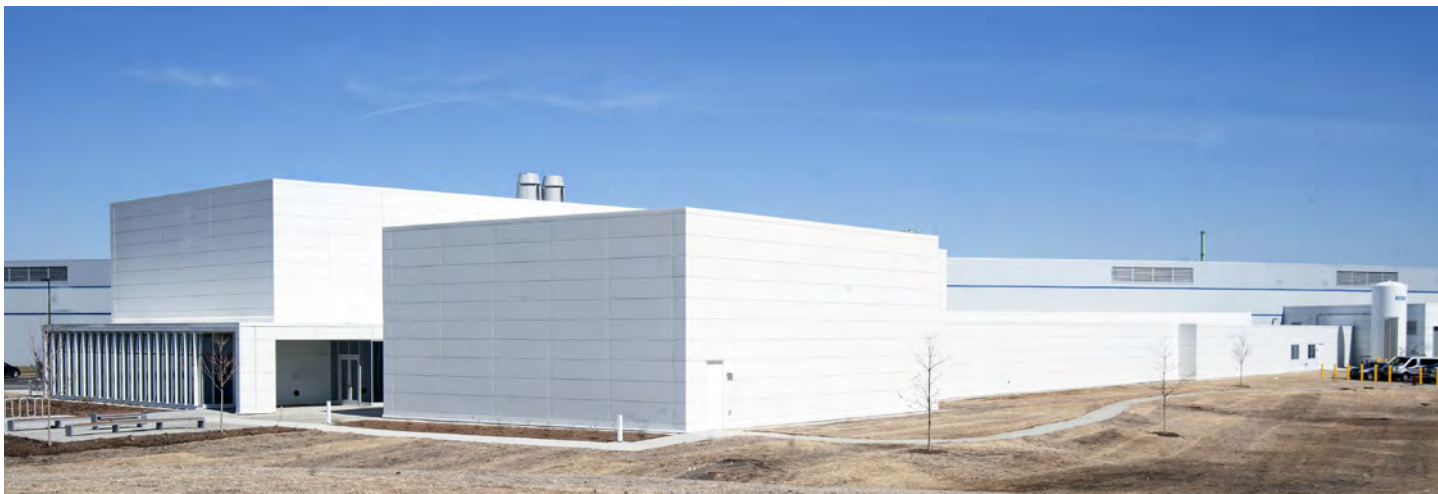
The Long Beamline Building, March 22, 2022.
