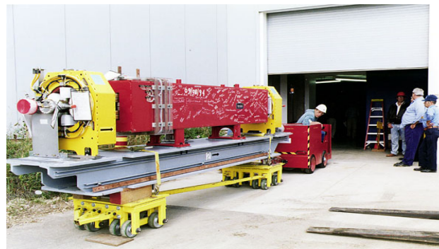
The last storage ring dipole magnet going into facility
