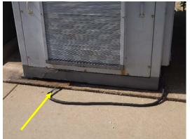
Fig. 1: Corrosion addressed with sealant paint on the RF3 matching transformer base.
