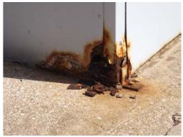
Fig. 2: Severe corrosion on the SG-R3 switchgear enclosure outside Building 420.
