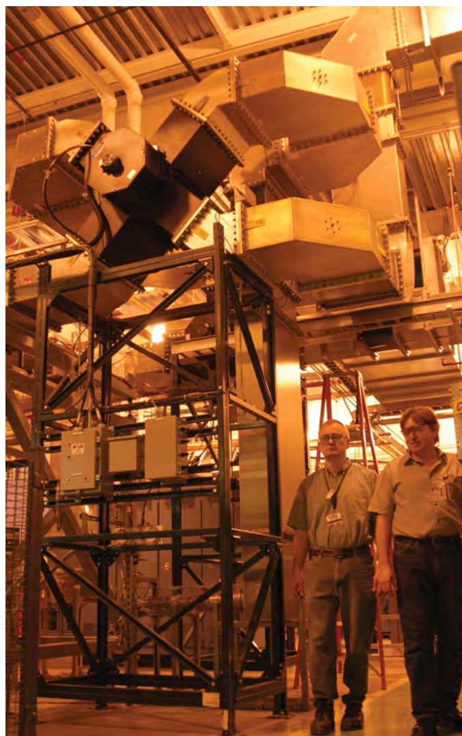
Fig. 5. Doug Horan (left) and Geoff Pile (both ASD-RF) walking under the rf waveguide switch #1.
