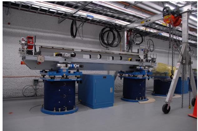
Figure 15: The first girder is shown installed in the LCLS undulator tunnel.
